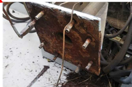
The situation of the back side of the signal column's base
