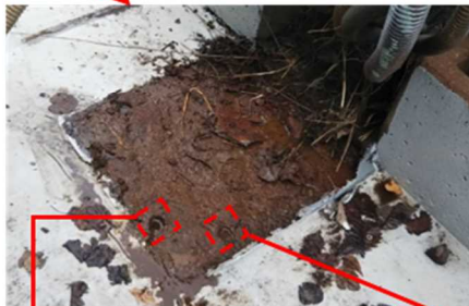
The situation of the concrete structure's surface
