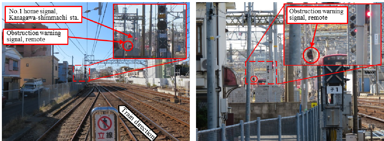
Figure 7. Sighting status of the remote OWS from the platform of Koyasu station
