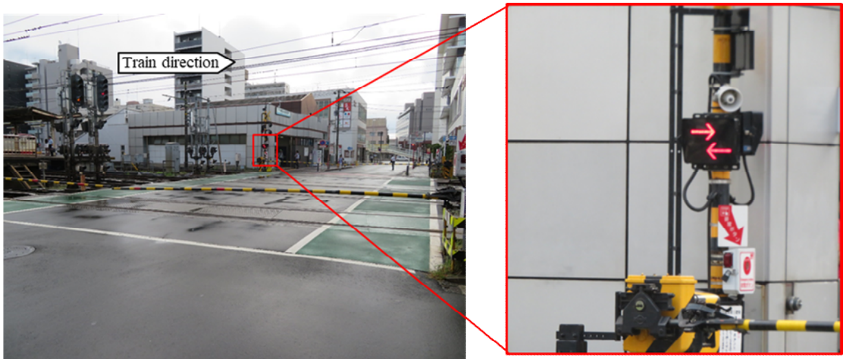
Figure 2. Train direction indicator in the Level crossing
