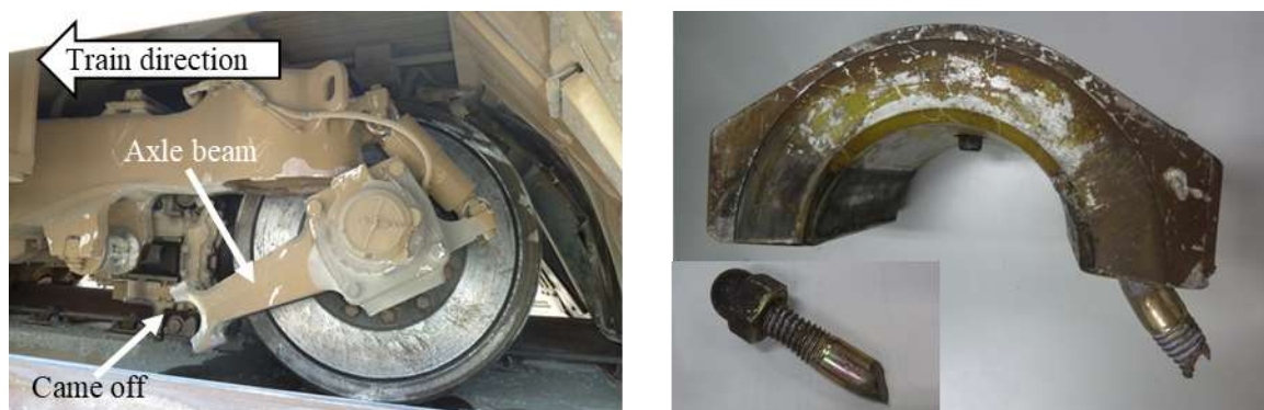
Figure 6. Damaged status of axle box suspension device, status at just after the accident in left, holding metal and snapped and broken bolt in right
