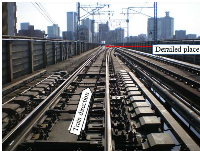
Photograph 2. Status of the Accident Site I
