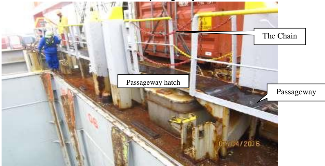
Photo 2 View of the passageway
