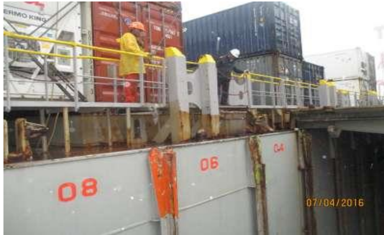
Photo 1 View of the area around the portside Hold No. 2
