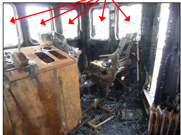
Photo ⑥ "Wheel House on Forward Starboard Area"
