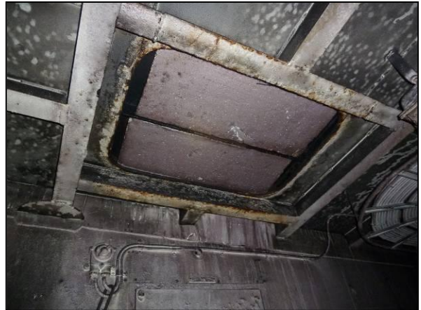
Photo 8 "Welded Escape Hatch on Upper Deck Ceiling"
