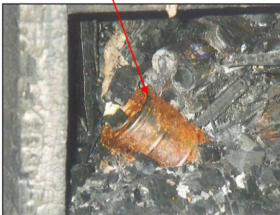
Photo ㉑ "Ashtray Found under Stairway"
