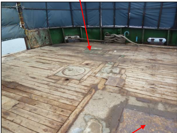
Photo 9 "Welded Escape Hatch on Quarter Deck"
