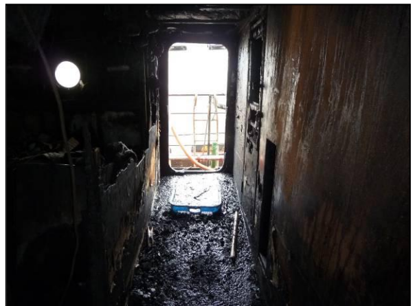
Photo 10 "Athwartship Corridor on Poop Deck"
