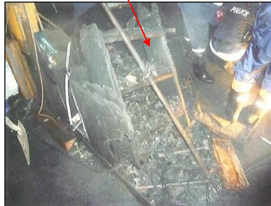
Photo ⑳ "Wooden Stairway to Fore Side of Bed of Ref/E"
