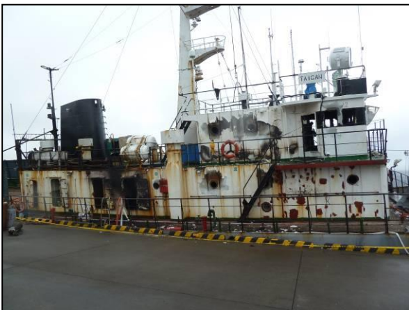
Photo 5 "Starboard Side of Accommodation Space Outer Plate"
