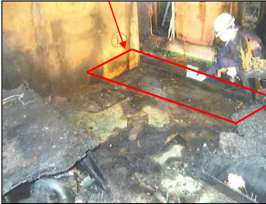
Photo ⑰ "Around Bed of Ref/E"
