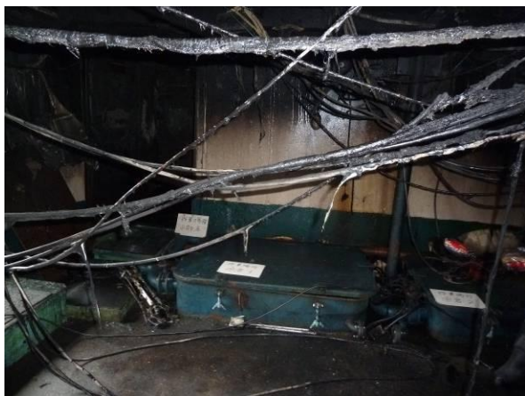
Photo ⑮ "Indoor Work Space 1)"
