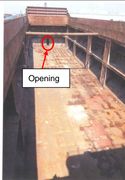
Photo 1. Cargo hold before loading
