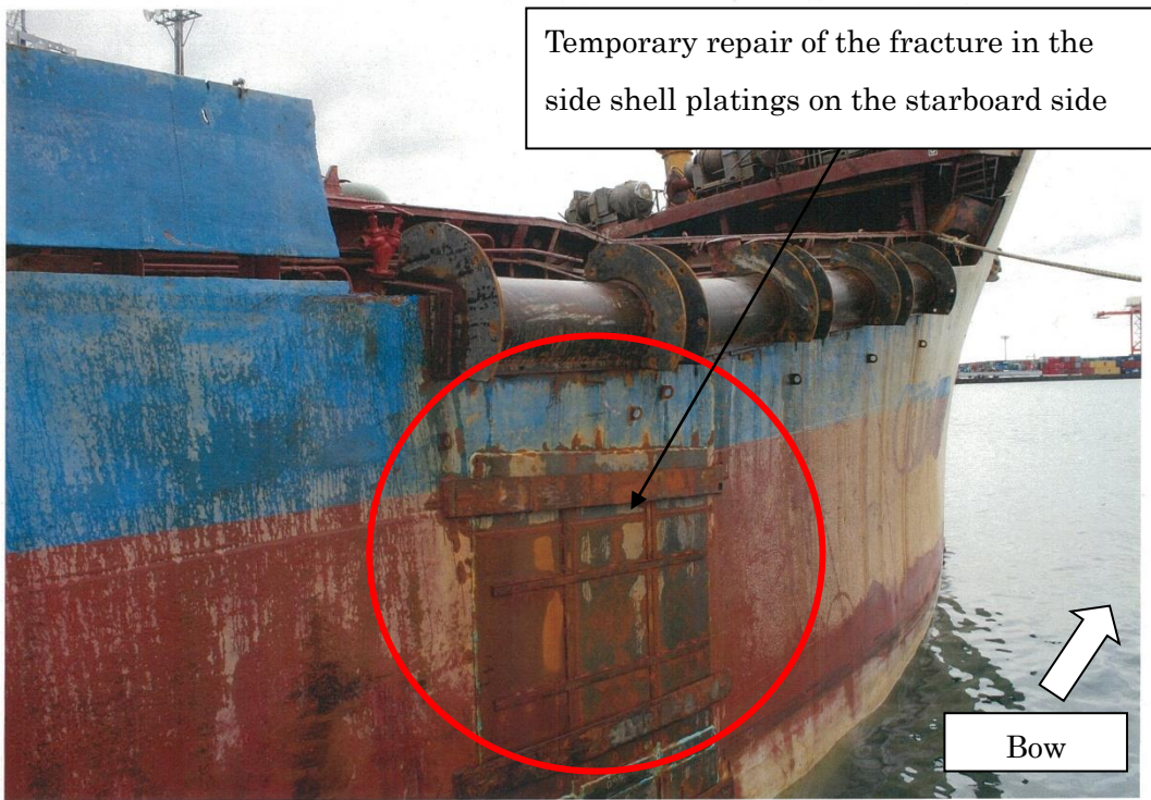
Photo 5 Damage to Vessel B (1) (Temporary repair of the fracture after being salvaged)
