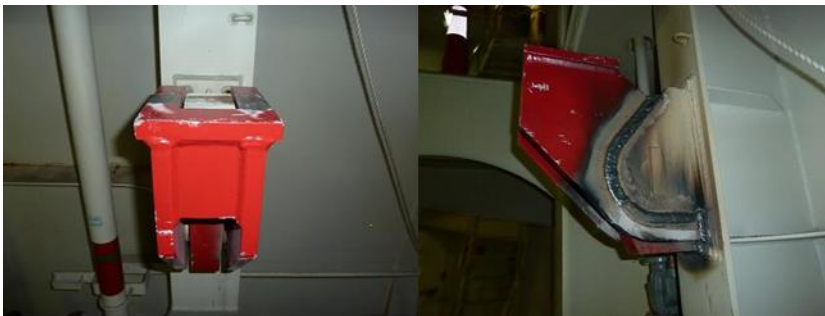
Photo 7.1: Improved Deck Support
