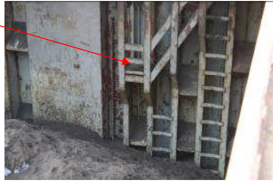
“Slanting Ladder on Aft-Bulkhead of Cargo Hold No. 3”
