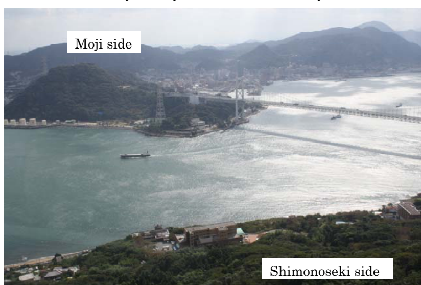
Vicinity of Hayatomo Seto Waterway
