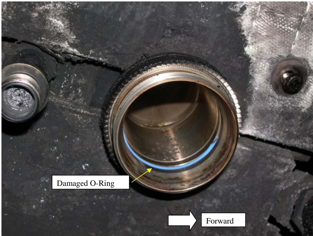
Photo 5 Fuel Supply Hose Coupling (Receiving)
