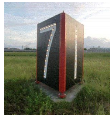
Photo 1 Runway Distance Marker Lights
