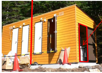
Photo 2.8 (1) Exterior of the toilet facility
