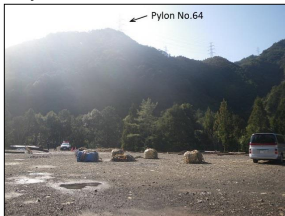
(Photo 8: View of Pylon No. 64 from the Forward Base (Photographed at 09:22, March 8, 2015))
