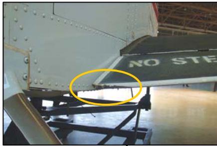
Damaged RH flap
