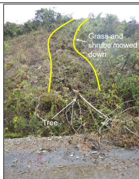
Figure 5: Slope viewed from below
