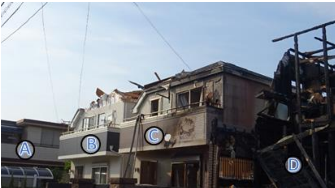
Photo 2.4.2-1 House A to House D
