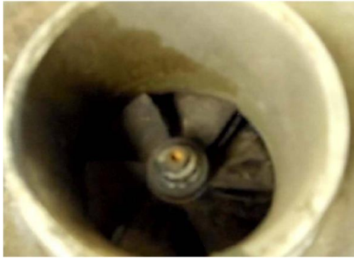
Photo #2 - Remains of compressor wheel
