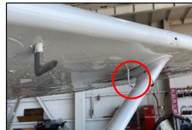
Figure 6: Fuel Tank Vent
