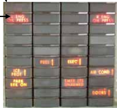
Central Warning Panel
