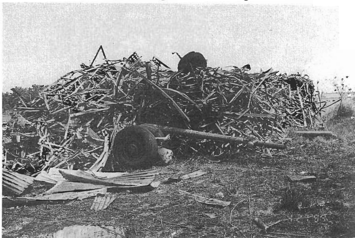
Photo.24 Tires of the Right Main Landing Gear
