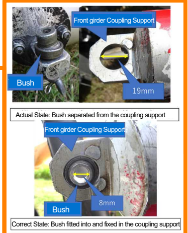
Fig. 5 Bush separated from coupling support of wing front girder due to wear
