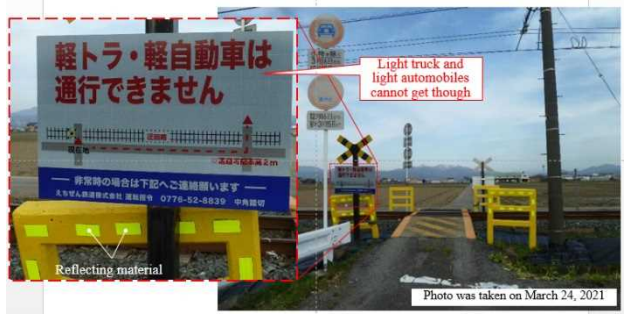
Figure Warning board planted by the company on the level crossing
