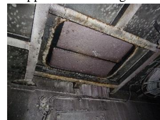
Welded Escape Hatch on Upper Deck Ceiling
