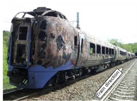
Status of the burnt cars
