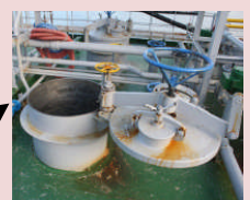
Manhole hatch of No.1 cargo tank on the port side
